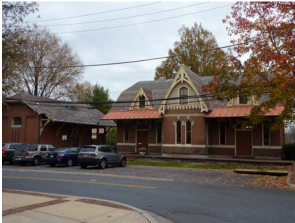
B & O Railroad Station 98 Church Street
